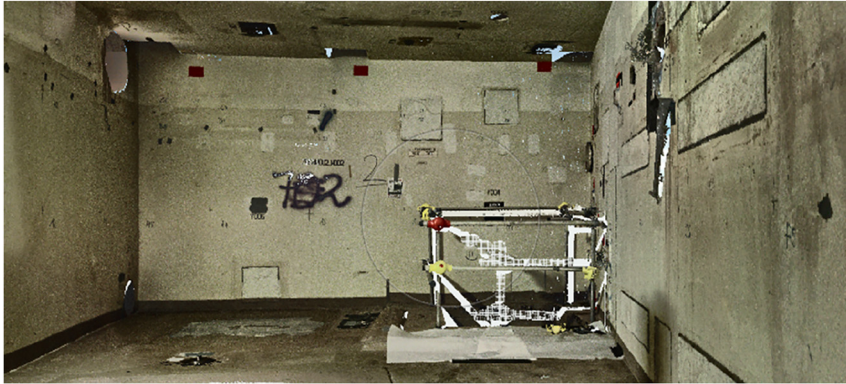
Figure 2: Detailed view of the point cloud of the building structures to be released in Mülheim-Kärlich.
